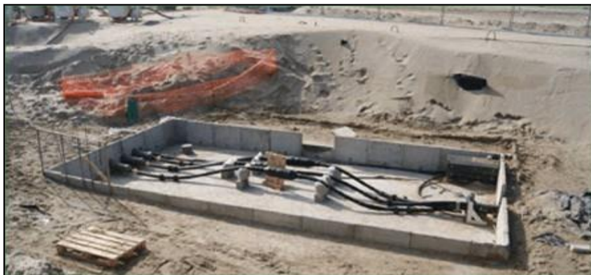
Figure 7: Landfall chamber under construction (RTE)
