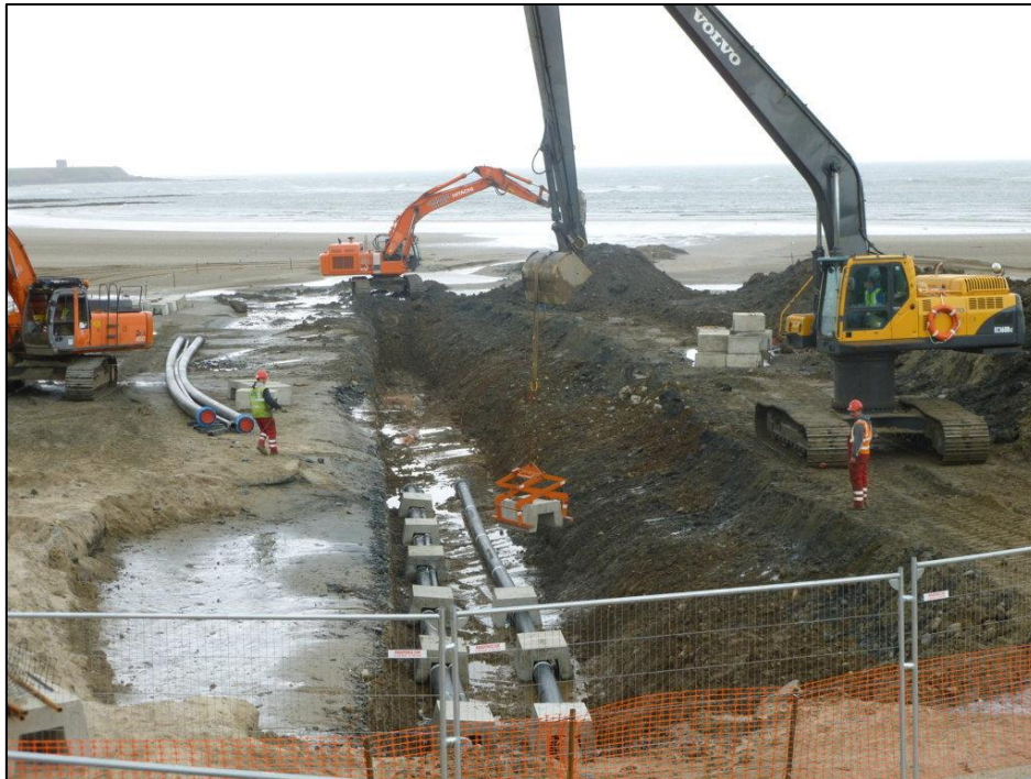
Figure 15: Example of an open-cut trench (source: EirGrid)
