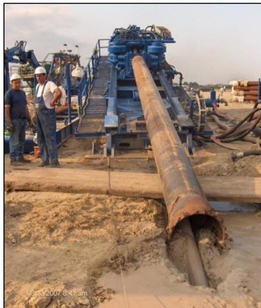
Figure 17: Directional drilling rig in operation
